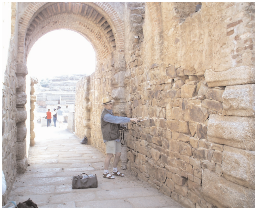
Figure 7. Sampling of mortar from the Roman amphitheater in Mérida helped to solve a mystery: Archaeologists had uncovered an inscription there indicating that the structure was erected in 7 BC; yet the similarity of this amphitheater with the 1 st -century AD Colosseum in Rome suggested that their construction was contemporaneous. Here mortar dating indicated that the amphitheater in Mérida was indeed built in the first century AD, indicating that the inscription represents older material incorporated into the structure by its builders.
